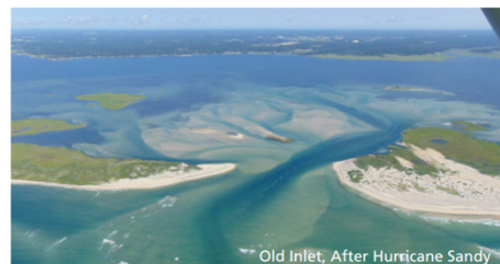
Old Inlet, After Hurricane Sandy
