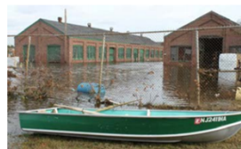
Maintenance facilities at Fort Hancock, located in the Sandy Hook Unit of Gateway National Recreation Area, were underwater and only accessible by boat after Hurricane Sandy.
