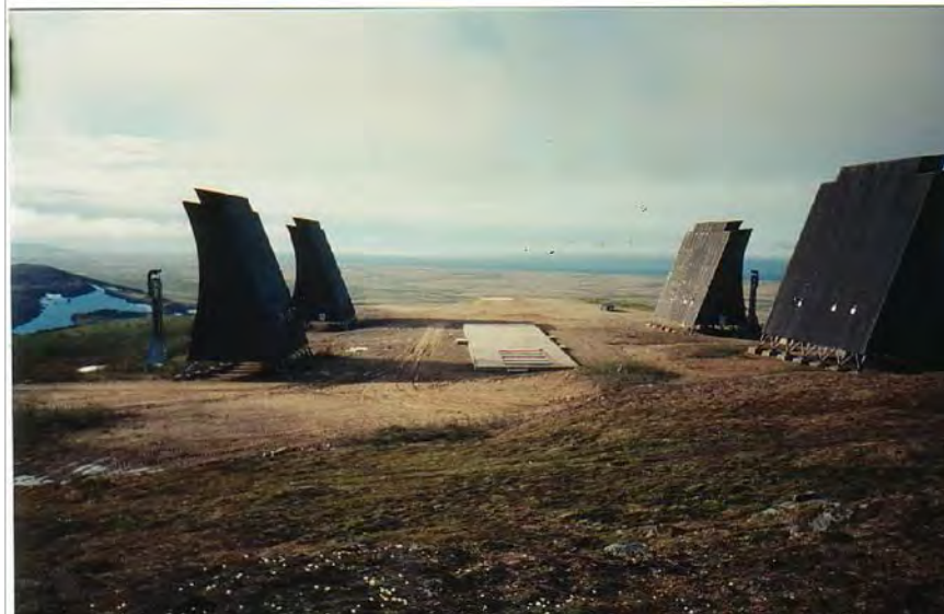
Figure H-135. WACS Tropospheric Antennas at the Former Anvil Mountain RRS Site
