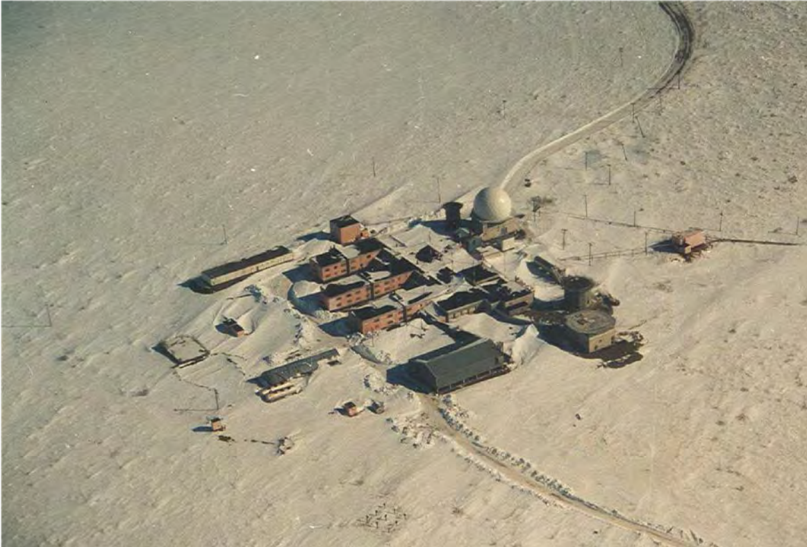
Figure H-75. Kotzebue LRRS, Prior to Demolition of Most Facilities
