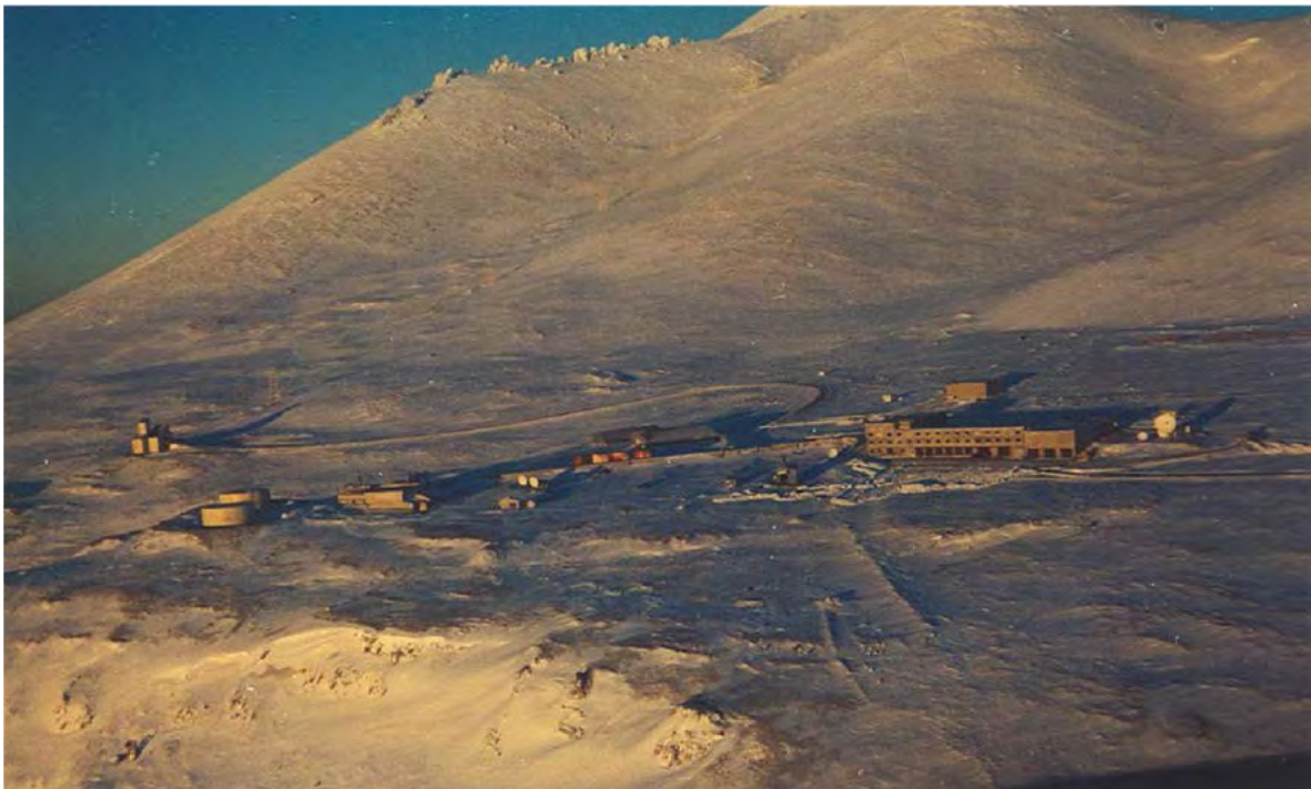
Figure H-109. Aerial Views of Tin City LRRS in the 1990s – Upper Camp (top) and Lower Camp (bottom)
