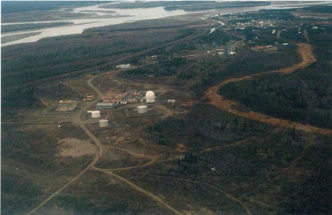
Figure H-64. Aerial View of Fort Yukon LRRS Looking Southwest
