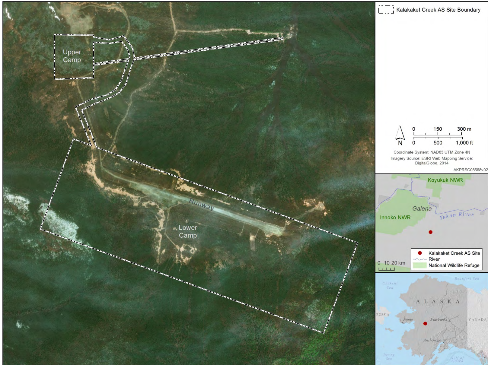
Figure H-160. Overview of the Former Kalakaket Creek RRS
