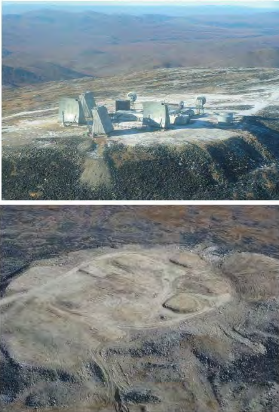
Figure H-157. Aerial Views of the Former Granite Mountain RRS, Upper Camp (before [top] and after [bottom] demolition)
