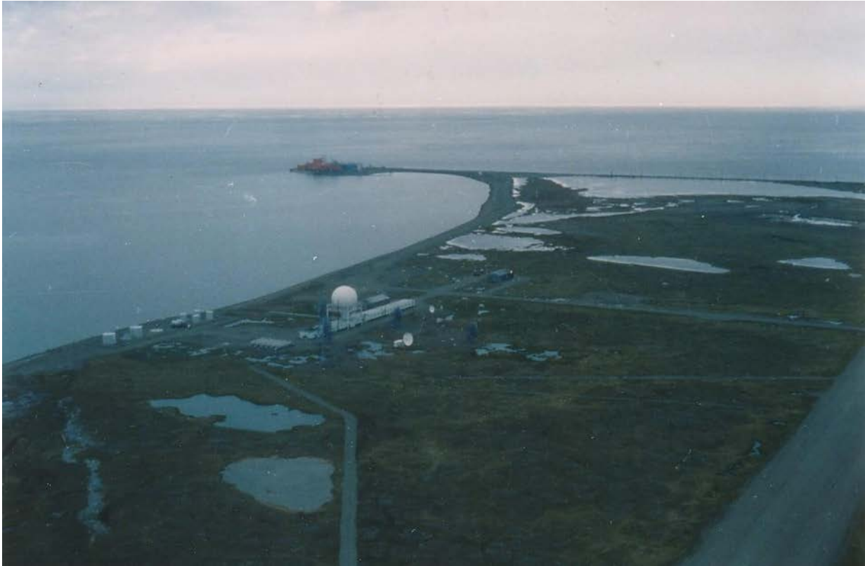
Figure H-85. Aerial View of Oliktok LRRS Looking Northeast towards Oliktok Point
