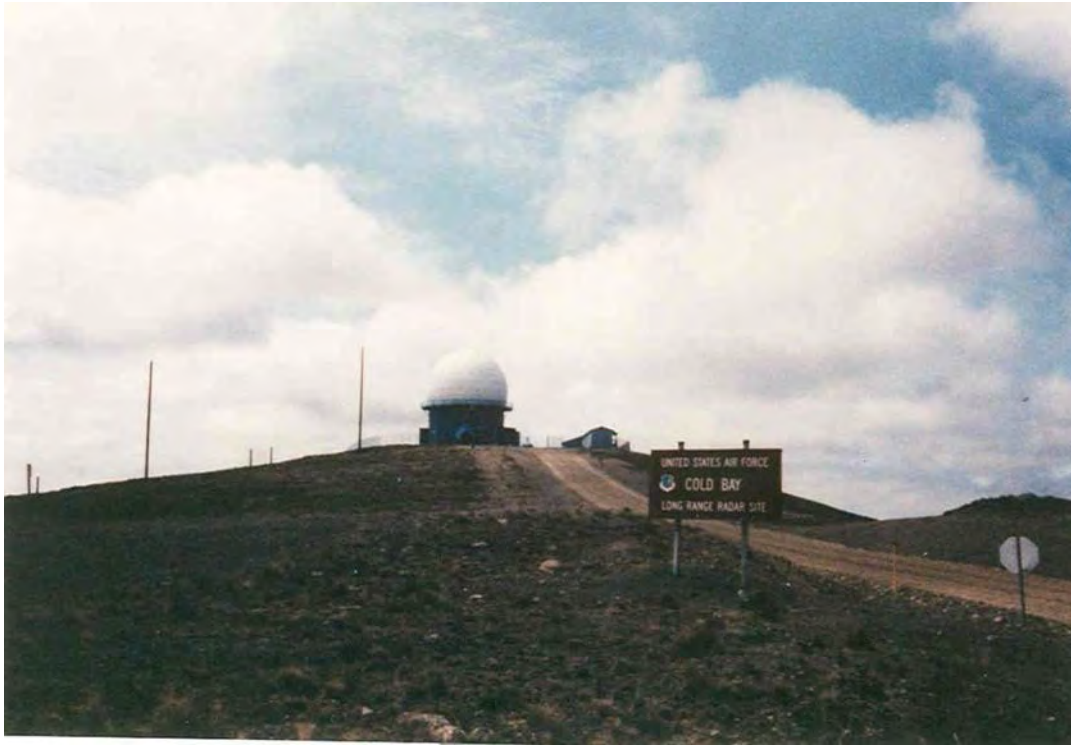
Figure H-55. MAR Tower at Cold Bay LRRS
