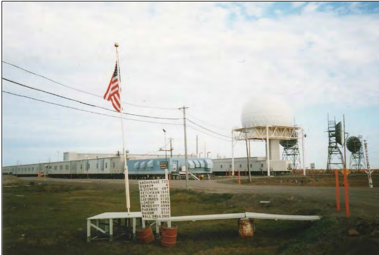
Figure H-92. Ground-level View of Point Barrow LRRS
