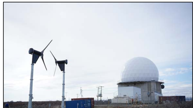
Rapidly Deployable Wind Turbine Project at Kotzebue LRRS (Photo: Capt. J. Goins, USAF)
